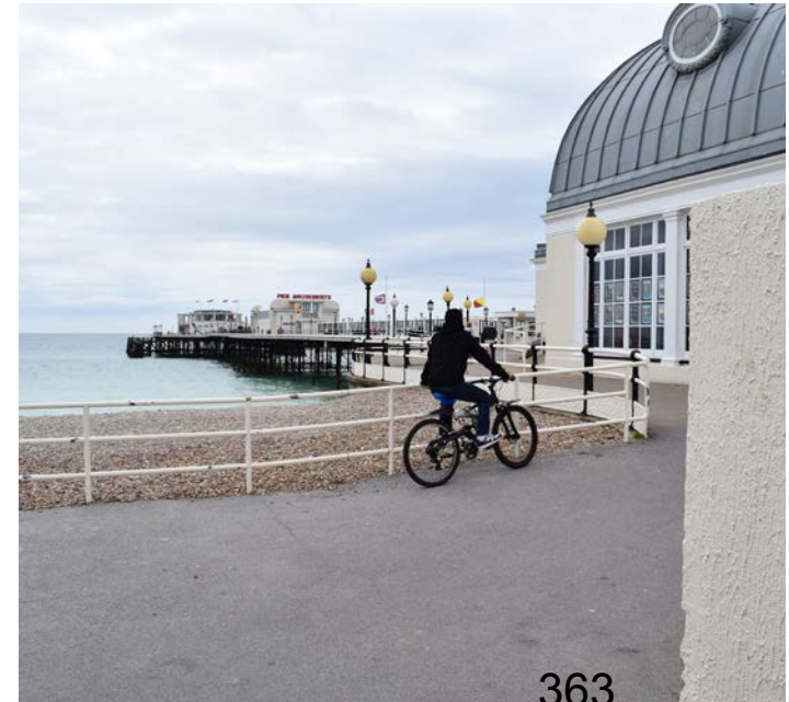
Access point to the Pier
