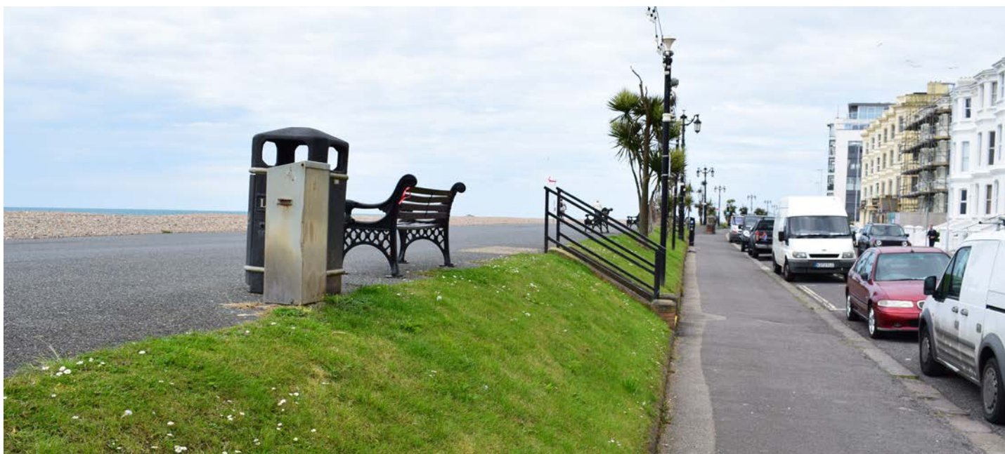
View showing change in levels on the promenade.
